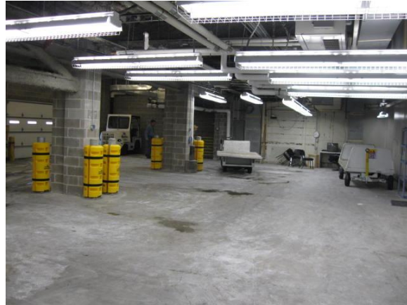
North end new lights, columns, protectors
